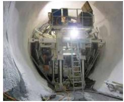
Full-round formworks are expensive to design and manufacture. The geometry and ring connector must be precisely adapted to the deformations of the concreting stage, otherwise it is impossible to strip the ormwork later on. With the full-round formwork of the new pumped storage power plant in Limmern, there was also the additional difficulty of gradients measuring up to 22 % and exceptionally tight spaces.
