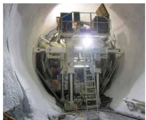
Full-round formworks are expensive to design and manufacture. The geometry and ring connector must be precisely adapted to the deformations of the concreting stage, otherwise it is impossible to strip the formwork later on. With the full-round formwork of the new pumped storage power plant in Limmern, there was also the additional difficulty of gradients measuring up to 22 % and exceptionally tight spaces.
